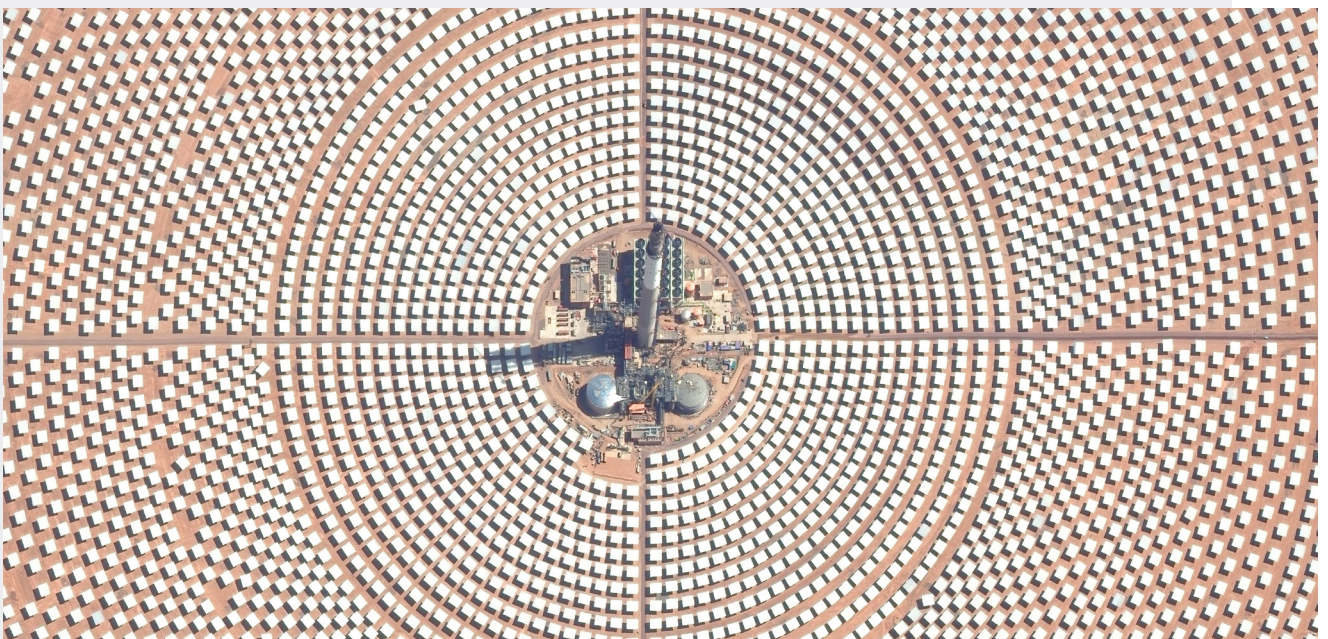
Satellite image of the Ouarzazate Solar Power Station. (Credit: DigitalGlobe/ScapeWare3d, Getty Images)
